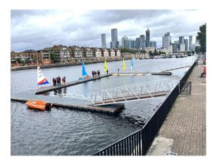
the pontoons have a low freeboard to assist disabled water sports users with embarkation and disembarkation to and from the dinghies and other watercraft. To meet this, Walcon created a new pontoon design that combines aluminium frames with low freeboard plastic floats that maintain the non-slip GRP grating deck at just 300mm above the water.
