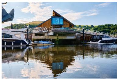
with special features that include premium fendering and extra wide central ducting along the back walkway for heavy duty cabling. The layout follows the line of the river, with finger pontoons replacing the previous alongside (two deep!) format.
