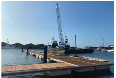
The design followed the original, three piers plus back walkway, configuration, but on a larger scale, A total of 32 fingers plus hammerheads created a total of 82 berths; 68 for Shoreham Port and 14 for the adjacent Sussex Yacht Club.
