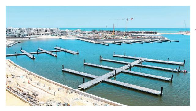
To add a touch of exclusivity, the five and tentonne cleats fitted to the pontoons are all Marassi branded. The marina is held in place by 186 steel piles, each protected from the sun and salt by HDPE sleeves and conical caps. Access to the docks is via 25, specially designed gangways, also decked in the walnut-effect, long lasting and environmentally friendly, WPC material.
