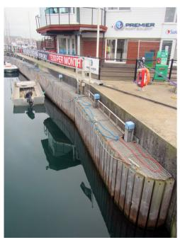
To ensure that the resulting top-heavy structure was stable required having pile guides at two levels. The space frames were helpful with this, enabling the positioning of the guides at the top and the bottom of the frames, far enough apart to provide the necessary stability. As an added benefit the solution also keeps the guides out of the water and so easier to maintain.
