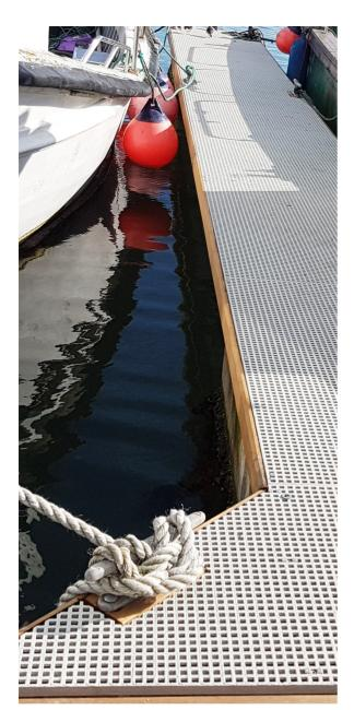
Over the course of eight weeks a Walcon team undertook the removal of the old decking and replaced it with a total of 910m<sup>2</sup> of heavy-duty mesh grating custom fabricated to match the exact dimensions of the pontoons. All this was done while ensuring that the resident fishing boats could continue to use the boat haven in their normal course of business.
