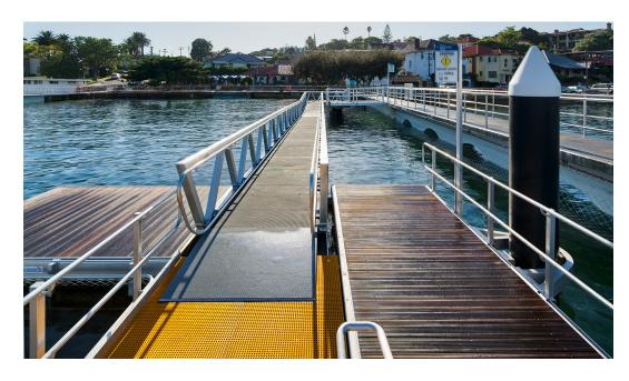
At the end of 2011 Walcon Marine was proud to complete the building and installation of the world's first, deep water 'Wheelchair Access Pontoon'. A specially designed and engineered marine pontoon, it has been created to allow the disabled and elderly wheelchair access into deep water, whether at pools, lakes or coastal locations.
