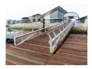
Another unusual feature is the bridge linking the shore to the marina. It is effectively fixed at each end to a section of decking that moves as a single piece as the walkway rises and falls in response to the tides. The decking sections attached to the head and foot of the bridge can move freely on hidden runners giving a smooth transition from shore to marina, free of obstacles, steps, or other hazards.
