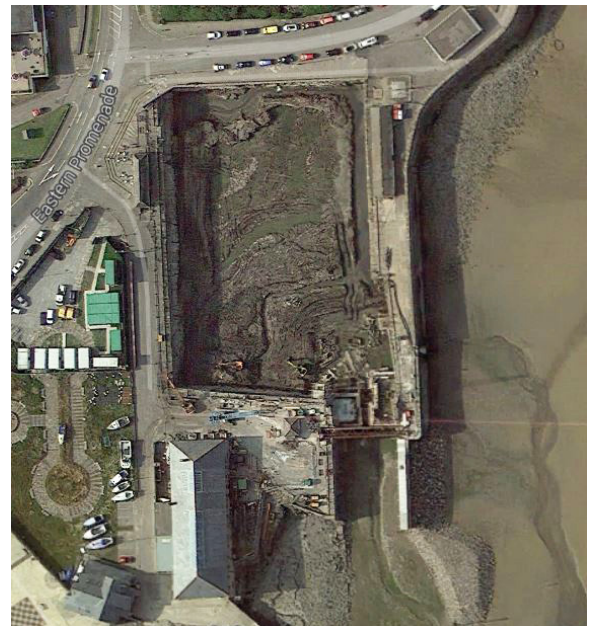
The Porthcawl basin undergoing initial works prior to the installation of the pontoons.
