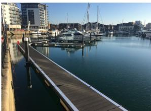
The new walkways, piers and pontoons were constructed using Walcon's proven and durable System 21 product range. For the decking, MDL specified a composite decking supplied by Dura Composites. A distinctive and attractive dark grey colour, it is extremely hard-wearing and has excellent non-slip characteristics as well as being visually appealing.
