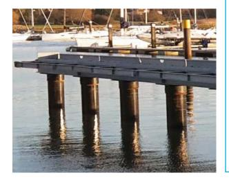
Whilst best known for its pontoons and marinas, Walcon also has a thriving civil engineering practice that enables it to undertake the design and build of marine structures such as hoist docks and breakwaters.
