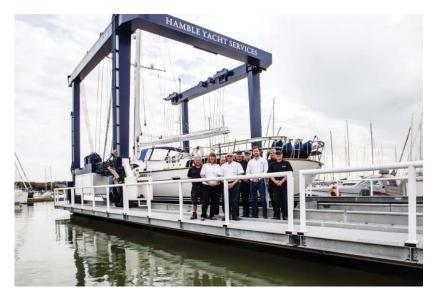
2017 Walcon Marine In completed the replacement of a travel hoist dock at Hamble Yacht Services (HYS) on the south coast of the UK. The company was responsible to every aspect of the project. It began with the demolition and removal of the old dock before moving on to the driving of new piles and the fabrication and installation of new steel runway beams followed by filling them with concrete.
